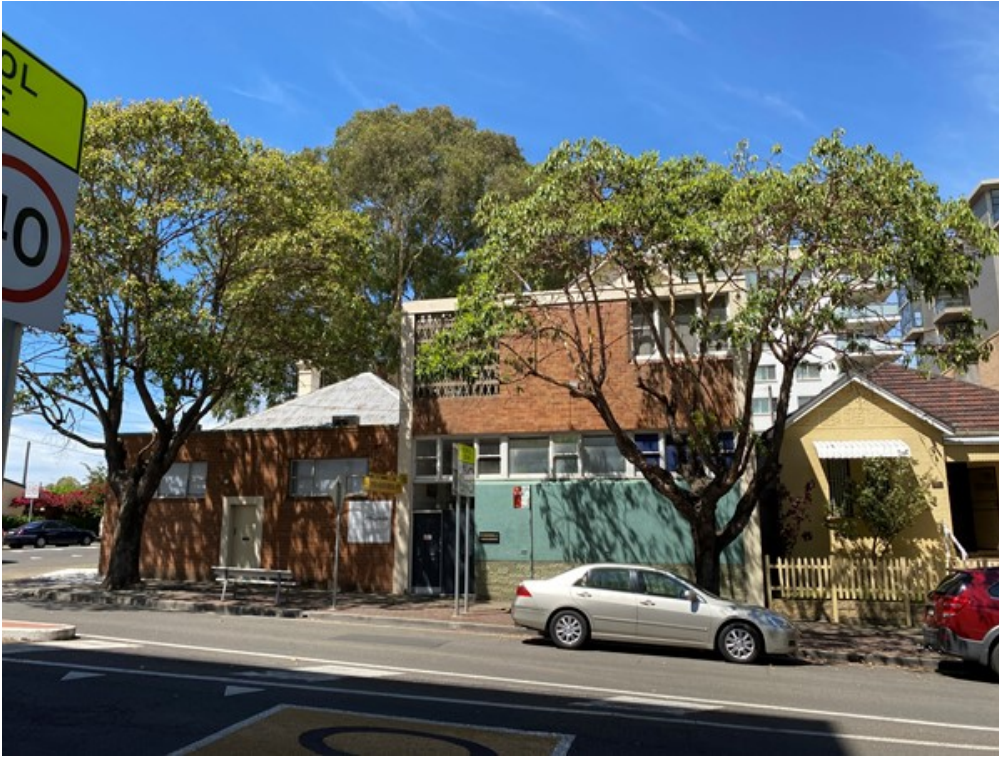
Figure 6: Subject site looking at the corner of King/George St
